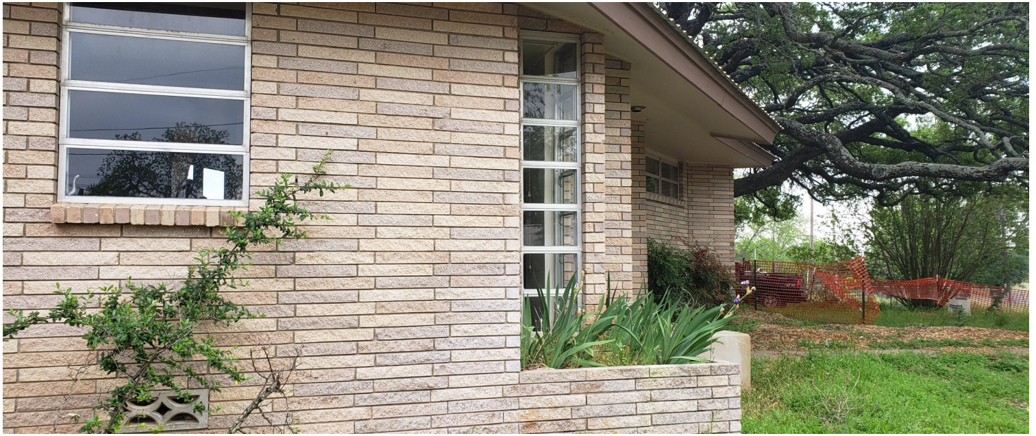
Side view showing acute angles created with windows and brick pattern
