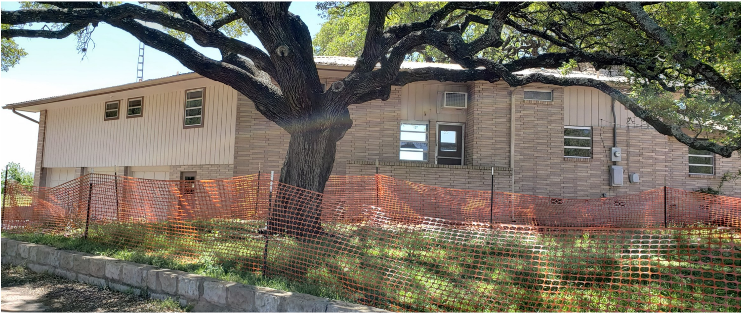
Rear elevation as seen from driveway
