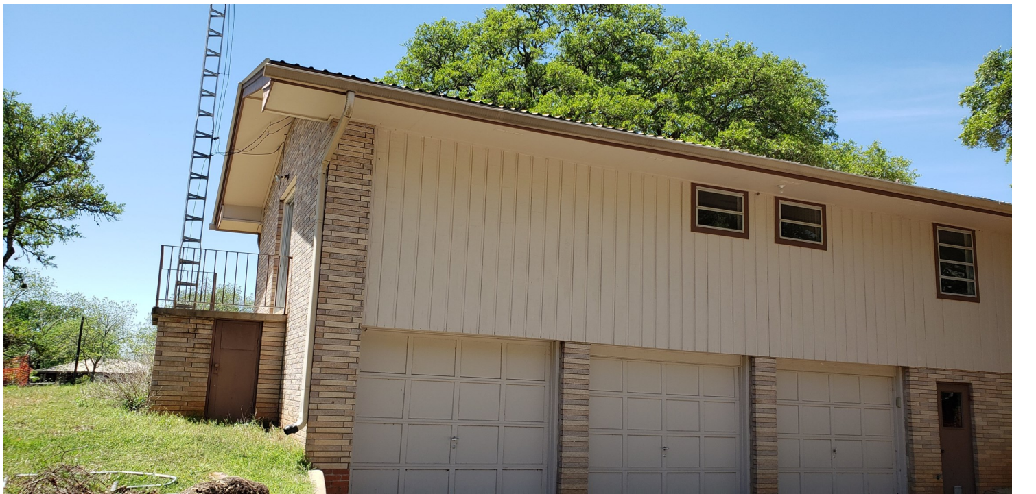
3 bay garage with bedrooms above V groove pine siding
