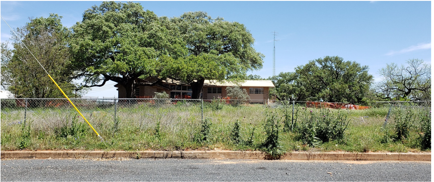
View from E Centre Street looking north
