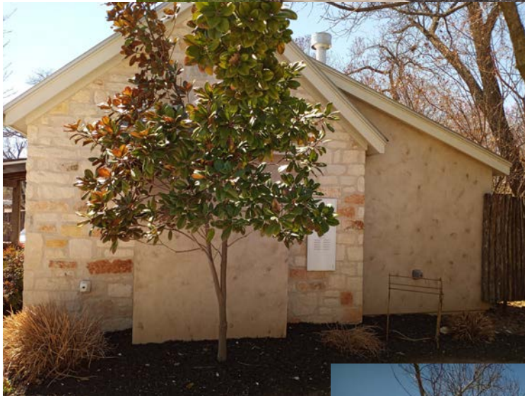
Existing 2 unit STR at 205 E Travis
