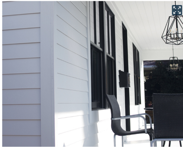
Lap Siding 6" Exposure Color to Match Mineral Paint Finish
