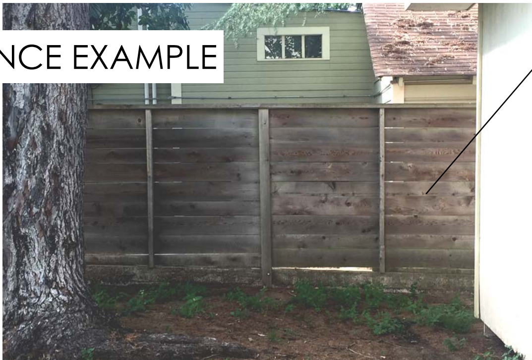
EXISTING SIDE PROPERTY PRIVACY FENCE LOOK TO REMAIN THE SAME FOR THE REMAINDER OF THE PRIVACY FENCE
