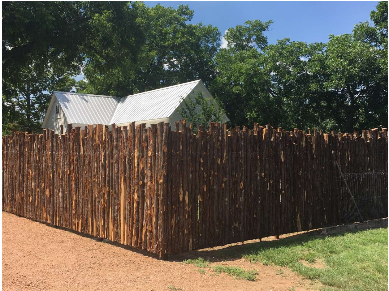
Existing view of SE corner of property from Driveway
