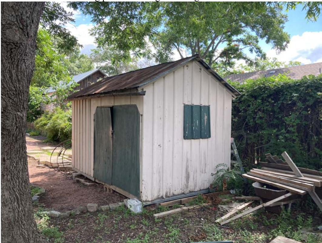
Existing portable storage building to be removed
