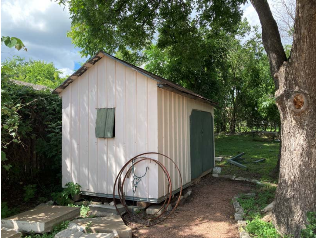
Existing portable storage building to be removed
