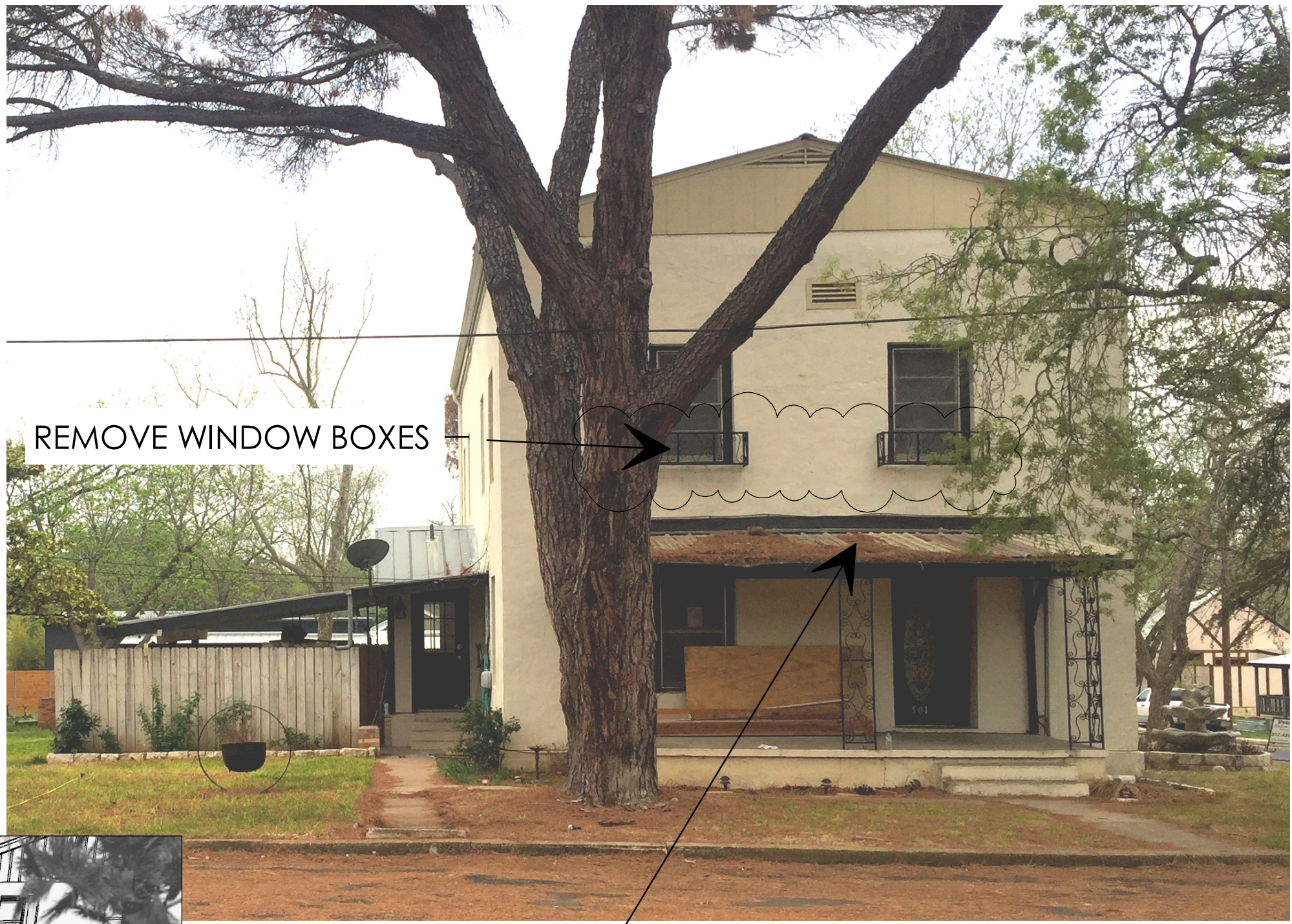
RE-ROOF THE ENTRY PORCH WITH GALVALUME STANDING SEAM EXISTING IS A SMALLER R-PANEL ALTERNATING WITH A WIDER R-PANEL SCREW DOWN ROOF
