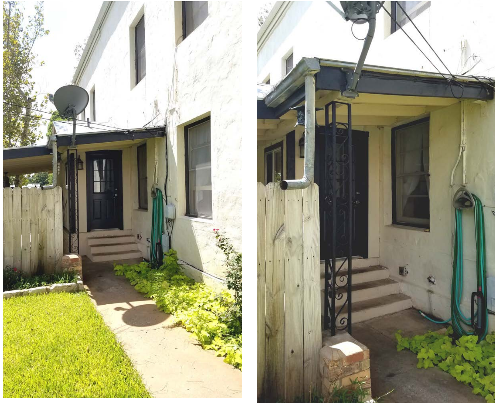
EXISTING PORCH VIEWS
