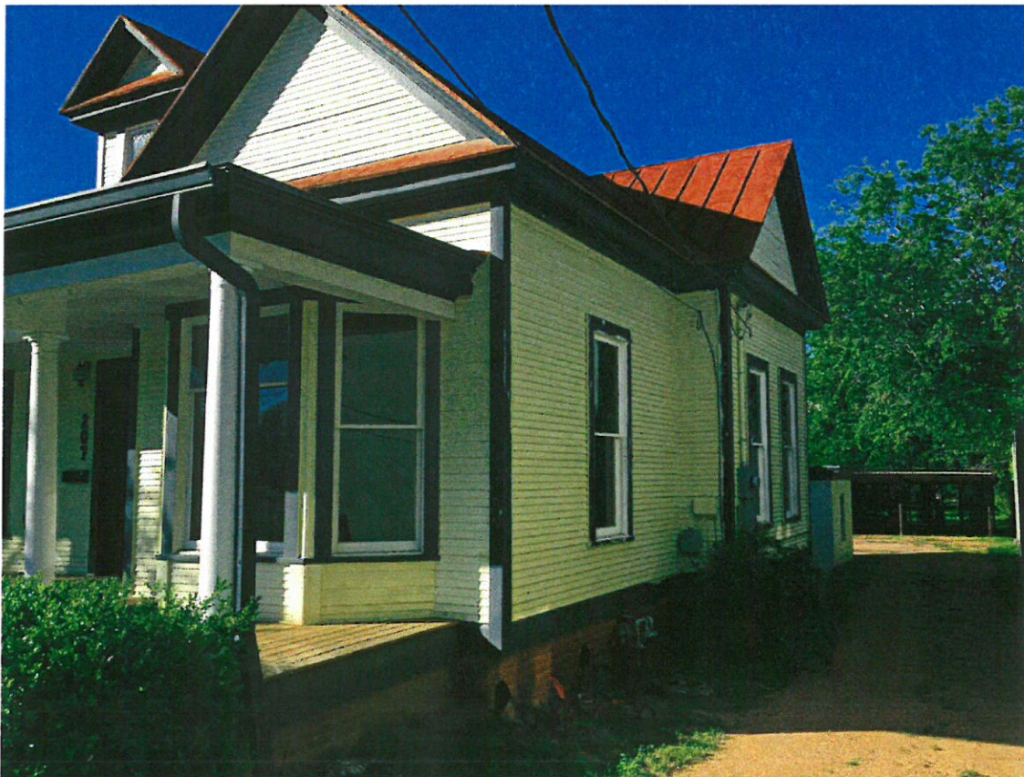
Northwest elevation (alley side)
