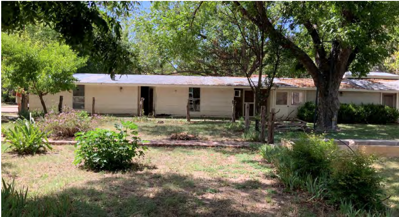
View from back yard looking west showing primary elevation of existing ADU
