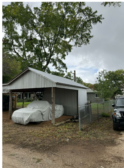
NEIGHBORING CARPORT AT ALLEYWAY
