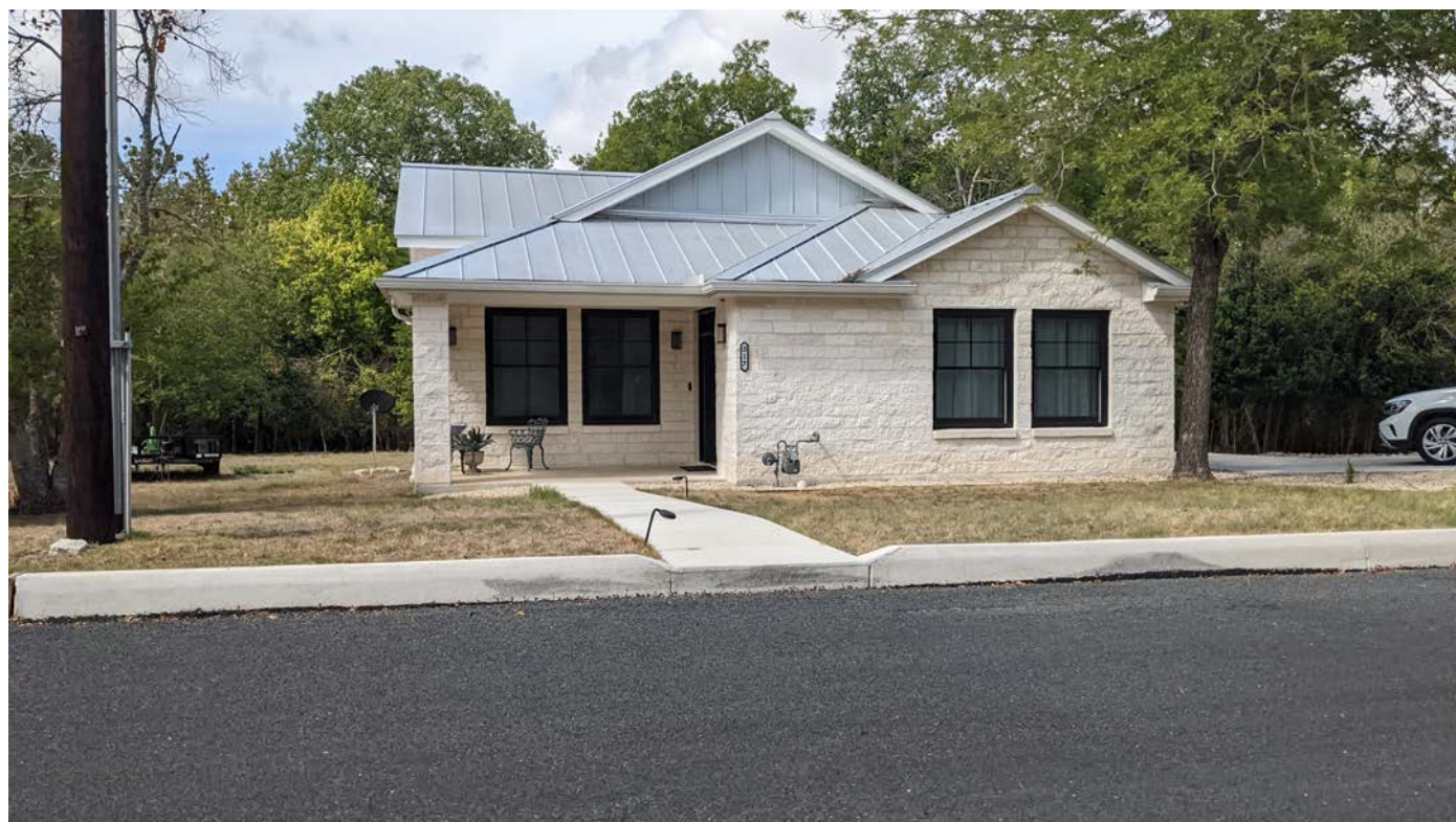
New construction to the west of empty lot.
