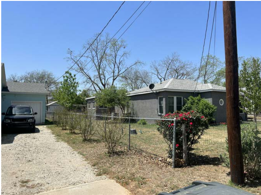
NEIGHBORING RESIDENCE TO WEST
