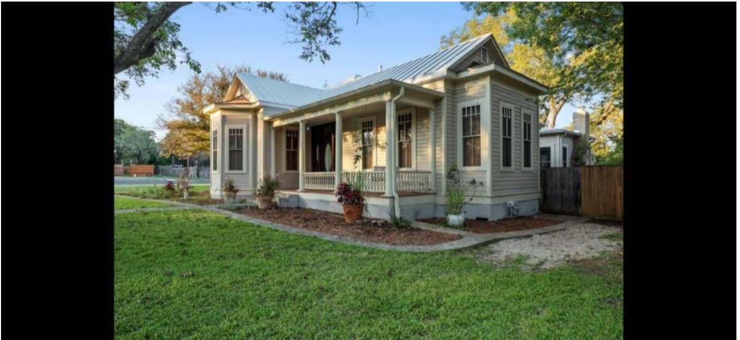
Photo 1. Oblique view from southeast corner of lot
