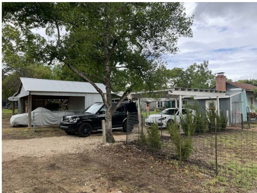
CARPORT AT ALLEYWAY TO BE REMOVED, NEIGHBORING CARPORT BEYOND
